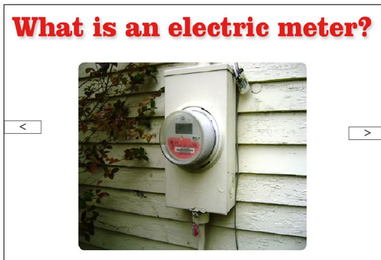
“Has anyone seen one of these on the side of a house or apartment building? This is called an electric meter. It measures the amount of electricity going into the building so the power company will know how much electricity has been used. Every month, people pay for the electricity they used.”
